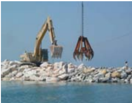
Excavator and grab barge placing rock offshore
