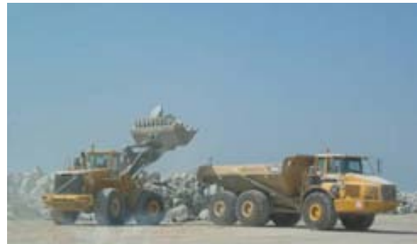
Loader rehandling armour to offroad dump truck
