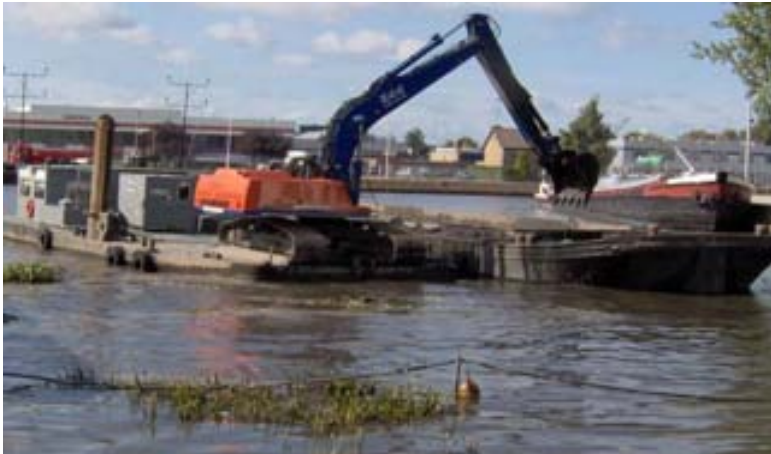
Figure 2-5 Typical backhoe dredge with split hopper barge being loaded
