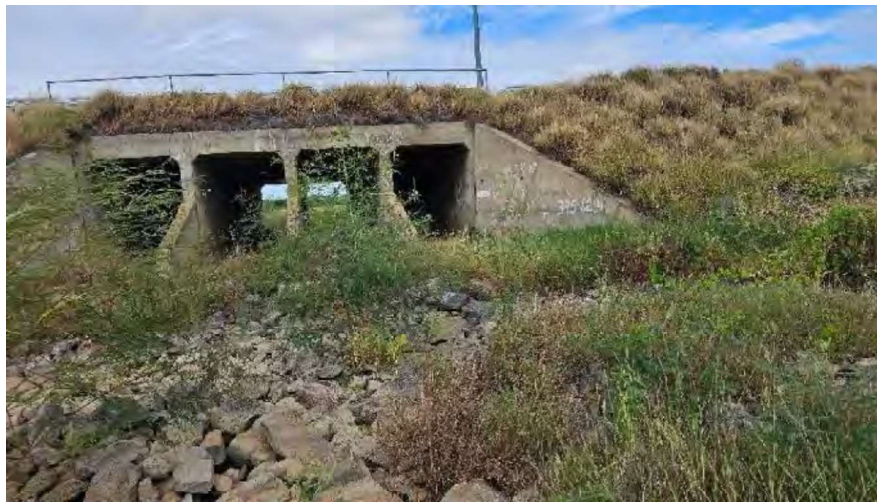
Photo 1 Culvert under the Mount Isa Line (photo provided by UGL)
