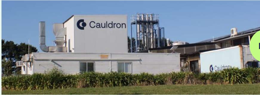
Hyper-Fermentation Demo Facility Customer pipeline, commercial demo
