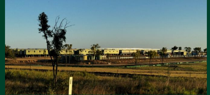
Construction Camp Site – 29/08/2024
