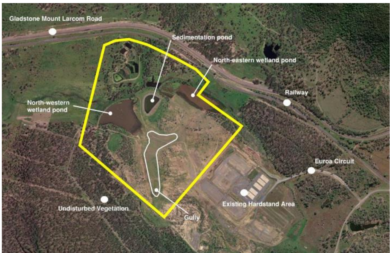
Figure 4-1 – Aerial View of Gladstone Manufacturing Hub Precinct (Yellow Boundary)
