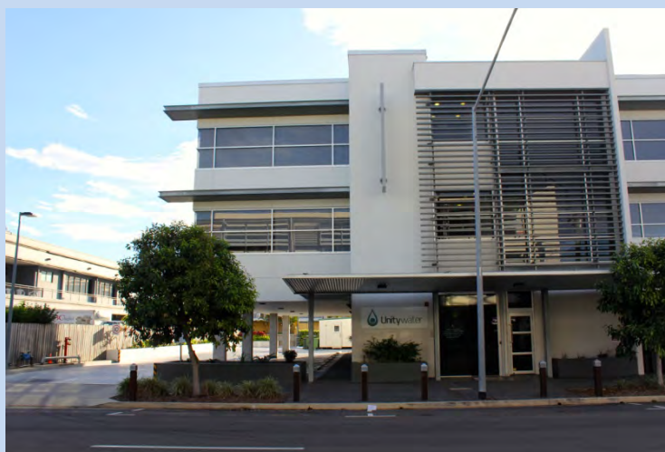
(Kawana) Screen at grade parking with landscaping to reduce visual dominance.
