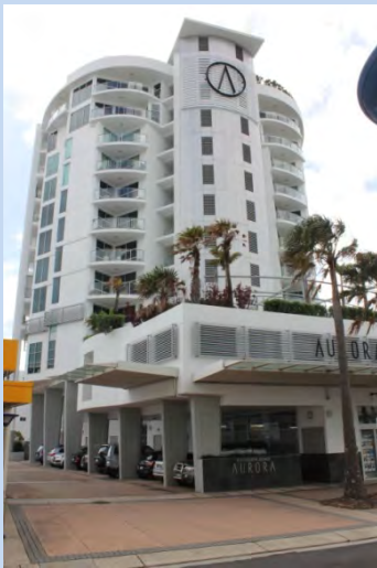
(Maroochydore) Screened at grade parking.
