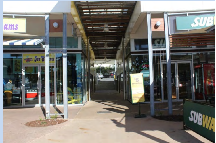
(Coolum) Access to rear car park from main street.
