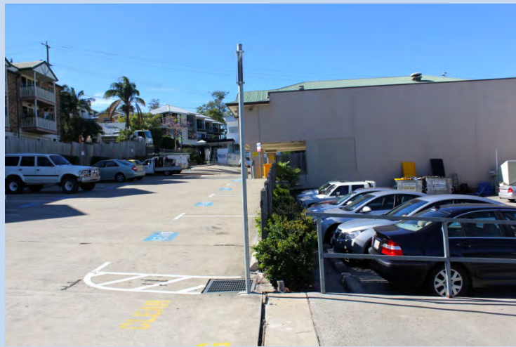
(Bulimba) Rear car parking area over looked by dwellings.
