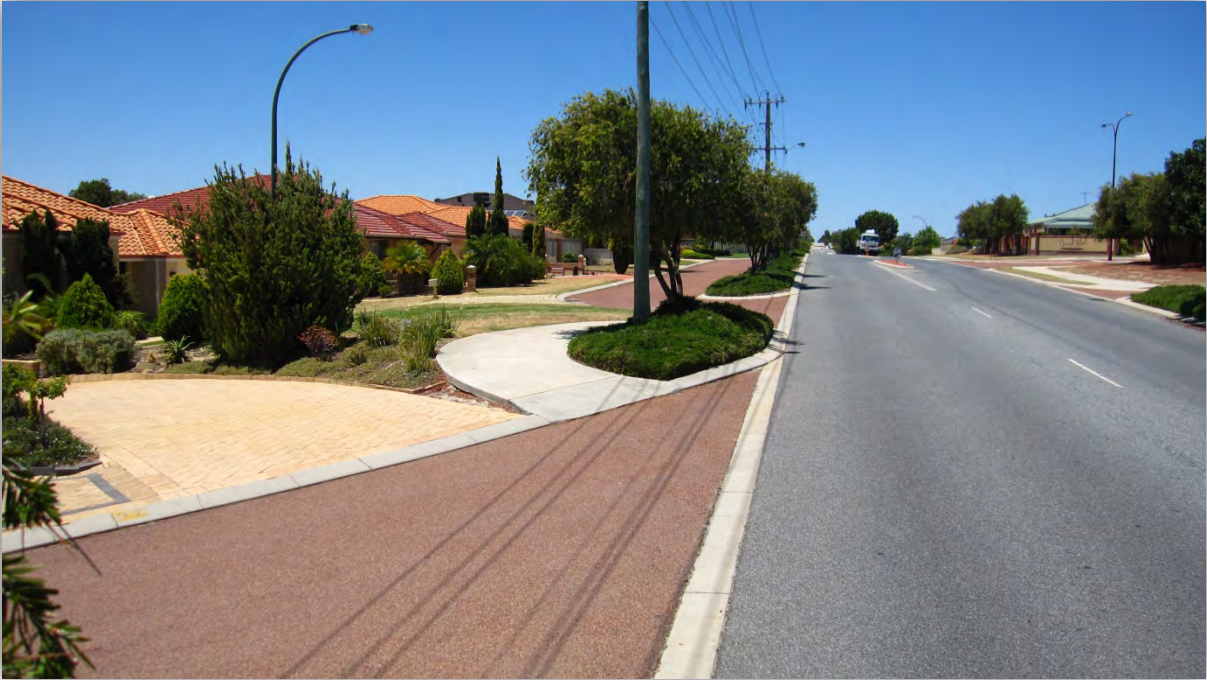
Higher traffic volume roads can still have frontage access by using innovative use of shared space and consolidated access
