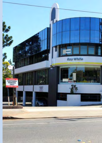
(Ascot) Using slope to reduce the visual dominance of at grade parking.
