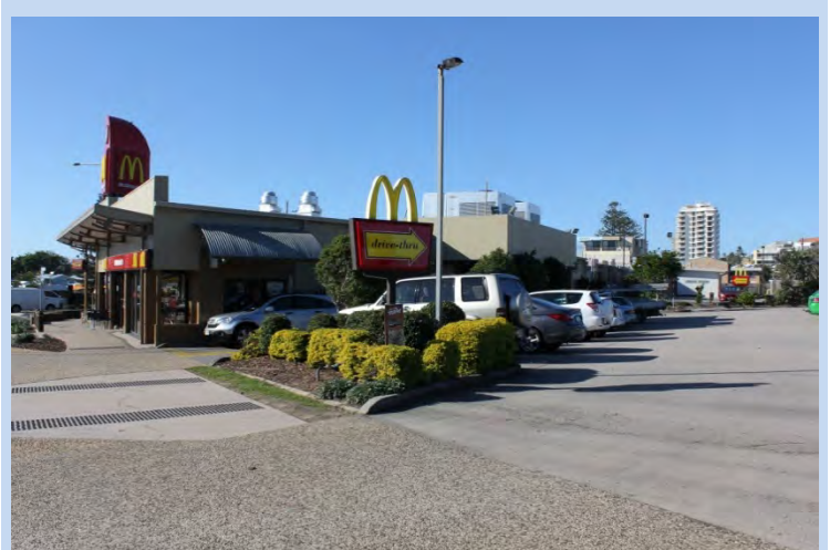
(Coolum) Drive through running behind the building not along the street frontage.
