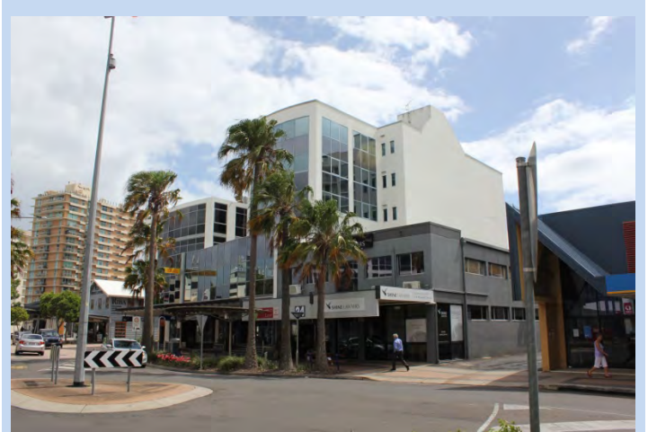
(Maroochydore) Shared driveway to rear servicing area.
