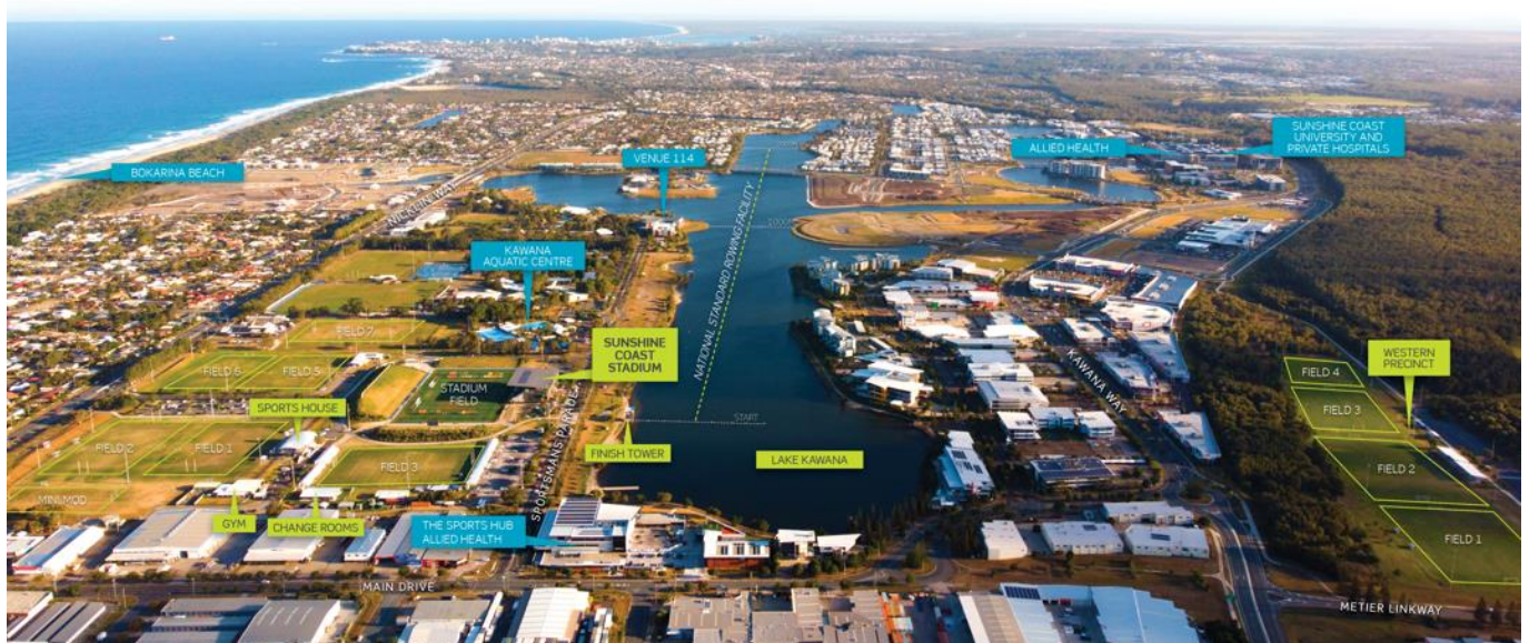
Figure 4: Location of the Sunshine Coast Stadium
