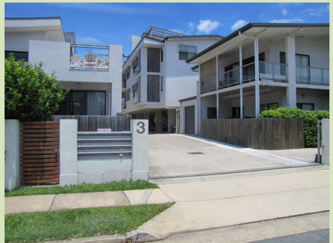
(Margate - Front view to see ground floor parking behind dwellings) The above example includes dwellings that adjoin and orientate towards the street with ground floor car parking located behind.
