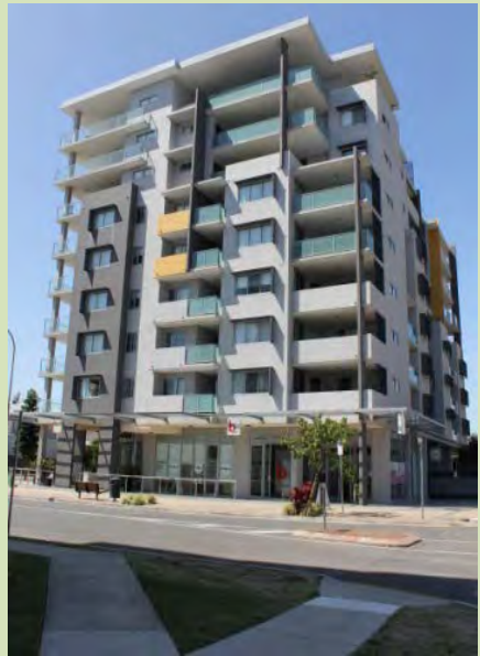
(Cherside) High buildings provide vertical articulation through a distinct top, middle and base section.
