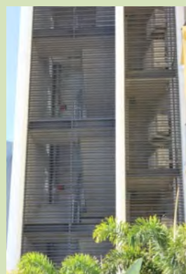
(Kawana) Screening of stairwells, and air conditioning units whilst maintaining ventilation.
