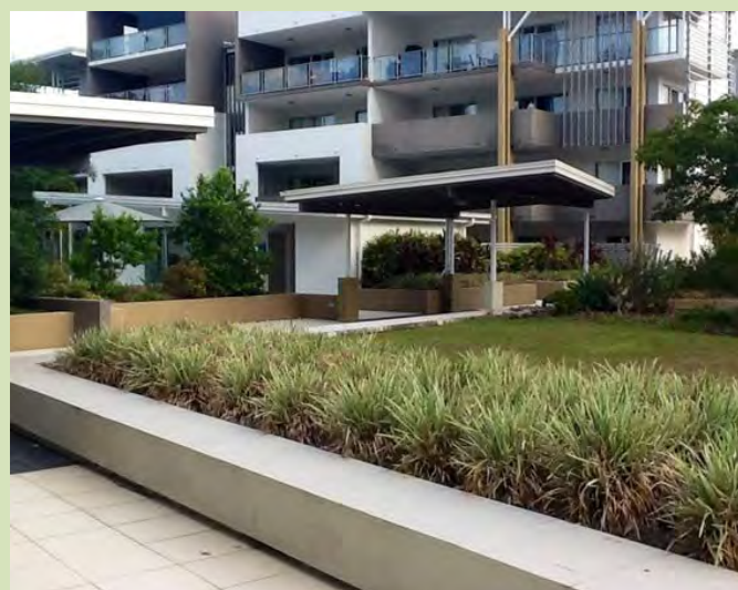
(Taringa) Solar access to communal open space should be maximised.
