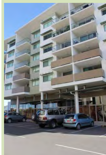
(Maroochydore) Solid balustrading for lower level apartments increases privacy while maintaining casual surveillance.
