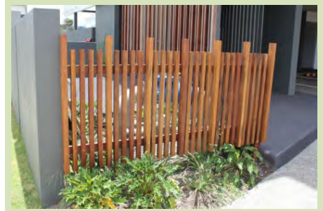
(Maroochydore) Semitransparent screening combined with landscaping can reduce the visual dominance of utilities while maintaining their visibility.
