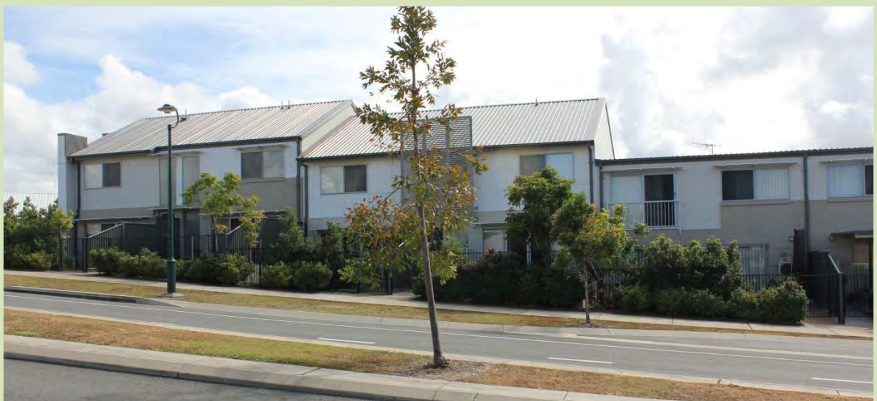
(North Lakes) Stepped terrace housing
