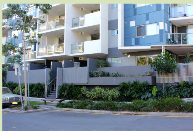
(Kelvin Grove) Where a retaining wall is unavoidable the height of the retaining wall and the fence should be combined and not exceed maximum fencing requirements. Additionally, the fence can be set back to allow low maintenance landscaping on top of the retaining wall in front of the fence.
