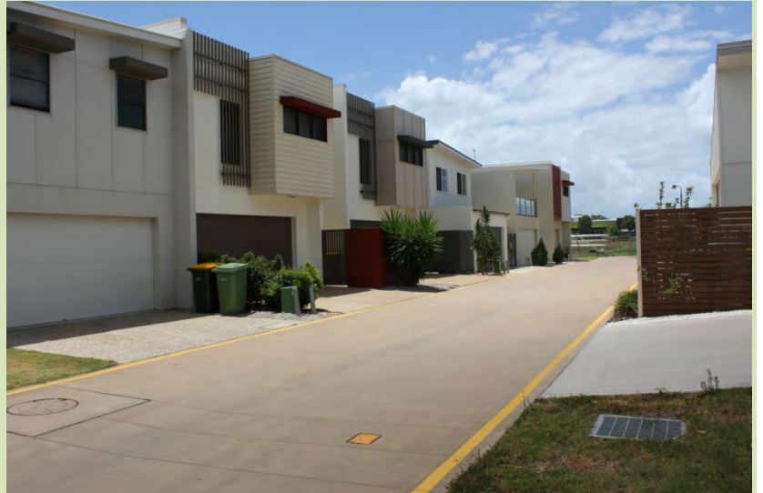
(Maroochydore) Rear – adjoining lane Lanes should reduce areas for concealment.
