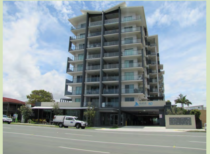
(Clontarf - Front on view to see screening treatments in effect) Mail collection, landscaping and an architectural feature forming part of the building all work together in this example to reduce the visual dominance of ground floor car parking areas.
