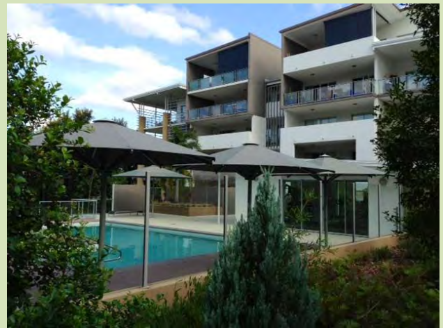
(Taringa) Communal open space should be easily accessible from the dwellings and other occupancies it serves and of a size and design suitable for intended users.
