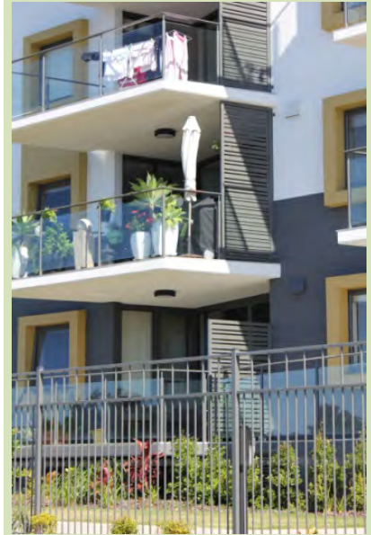
(Kawana) Where balconies are used to house equipment and plant such as clothes drying, air conditioners etc. this equipment should be screened.
