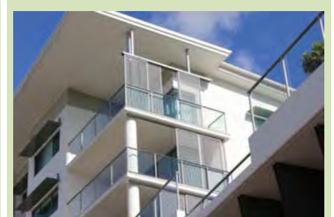
(Maroochydore) design solutions such as louvred screens with specific views, operable or fixed vertical louvres or planter boxes along the edge of balconies should be utilised to limit sight lines. Obscure glazing is the least desirable screening method for apartments.
