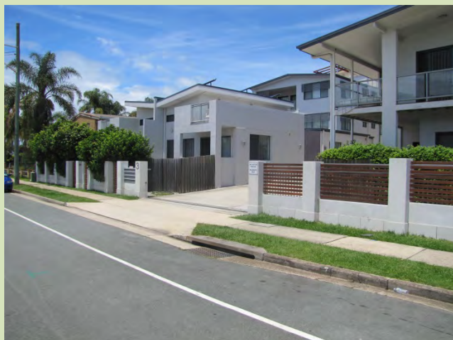
(Margate - Angled side view to see dwellings adjoining the street) The above example includes dwellings that adjoin and orientate towards the street with ground floor car parking located behind.
