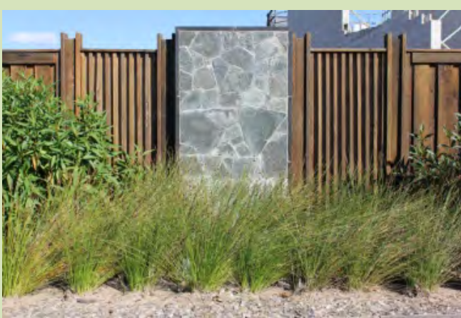
(Maroochydore) Where solid fences are unavoidable they should include variation in material, reduce flat surfaces and incorporate landscaping in front to reduce visual dominance and assist in the prevention of graffiti.
