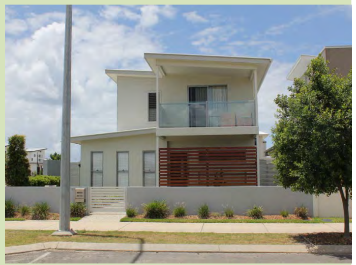
(Maroochydore) Garages adjoin a lane ensuring they do not dominate the streetscape.
