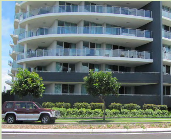
(Suttons Beach) The above example utilises a combination of landscaping and solid rendered balustrade to reduce the visual dominance of a protruding basement.
