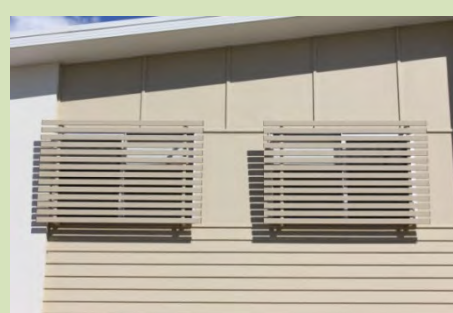
(Maroochydore) Fixed screening over windows is not a desirable solution to overlooking as shown above. Windows should be offset or have an appropriate separation distance.
