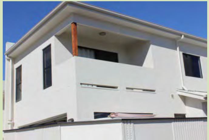
(Maroochydore) Solid balustrading can provide privacy to balconies whilst also facilitating surveillance.
