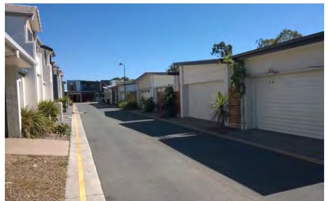
Laneway Houses (Front and Rear) (Fitzgibbon Chase)
