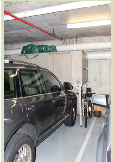
(Maroochydore) Storage above car bonnets should not be the only storage provided for occupants.
