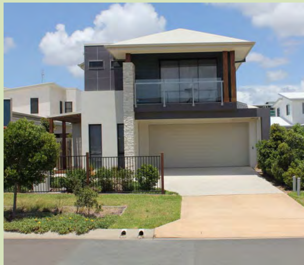
(Maroochydore) Garages and car ports are to be setback from the frontage to reduce the visual dominance on the streetscape and allow tandem spaces for cars
