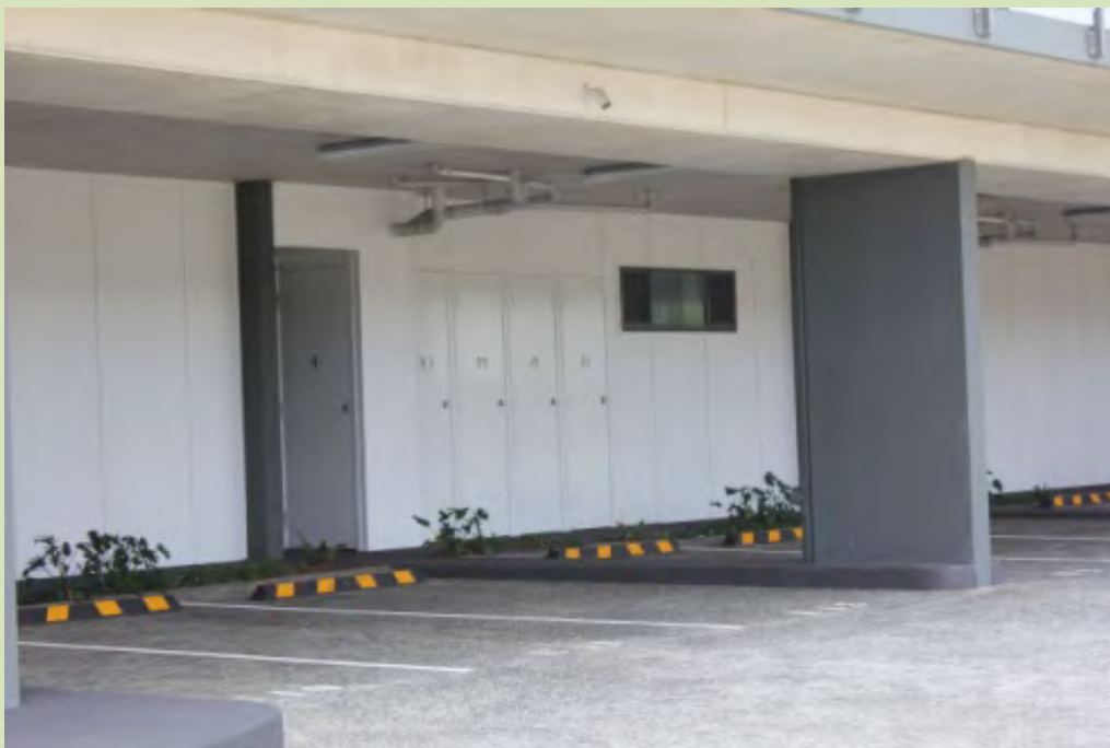
(Maroochydore) Each dwelling should have convenient access to secure storage. Storage spaces should be clear of any services and other obstacles.
