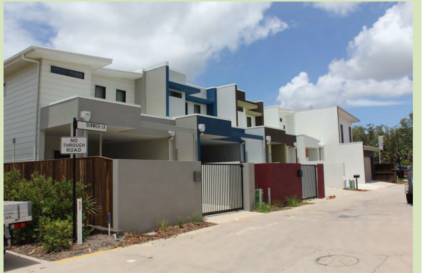
(Maroochydore) Rear – adjoining lane Fencing to a lane can be 1.8m high and 0% transparent to screen private open space and servicing areas.
