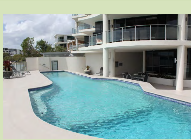
(Maroochydore) Communal open space must be usable and provide reasonable levels of amenity.
