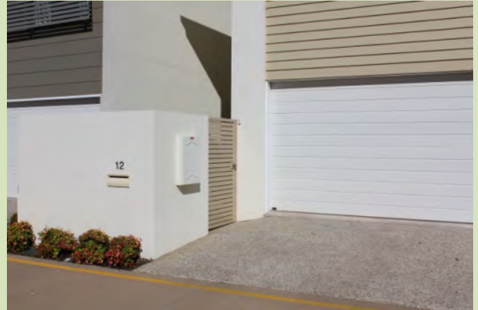
(Maroochydore) Visual clutter created by utilities should be screened in laneways.
