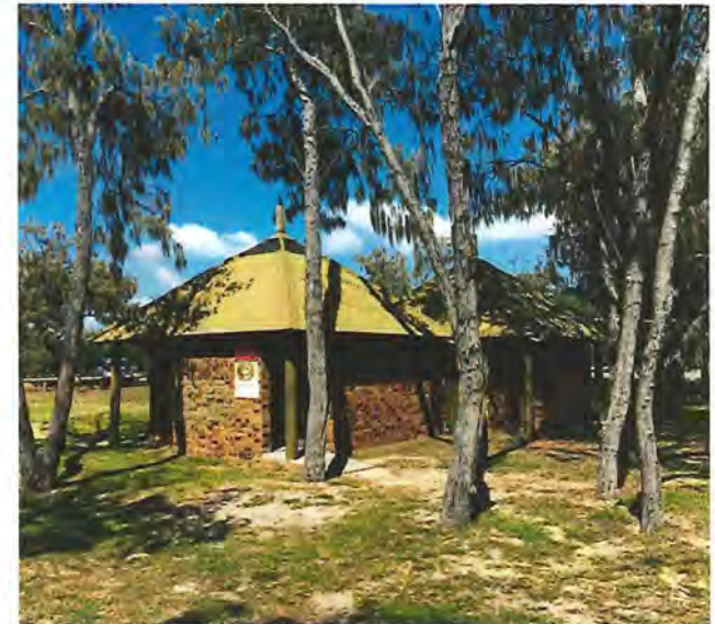
Figure 5.10. Philip Park toilet block
