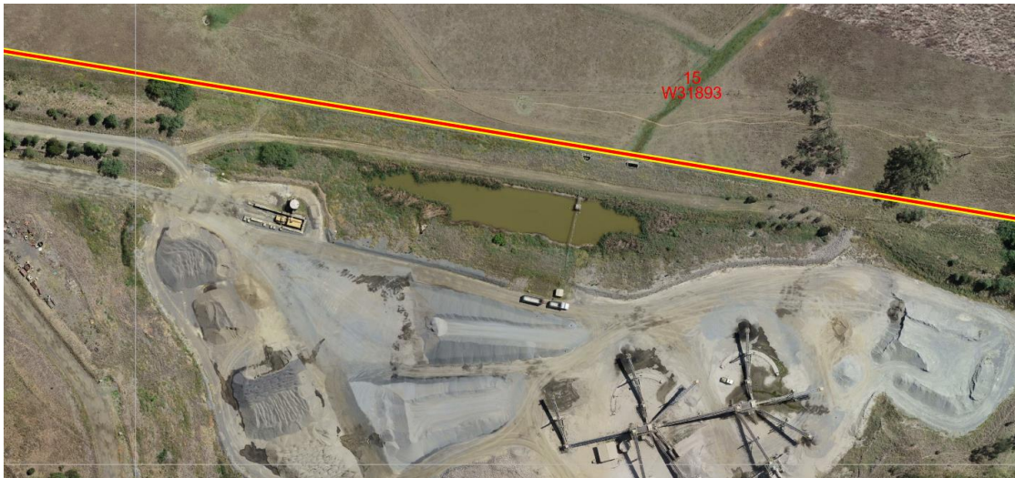
Plate 6: Processing Plant and Operations Area
