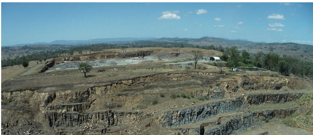
Plate 8: West Pit landslip with Adjacent Quarry in background
