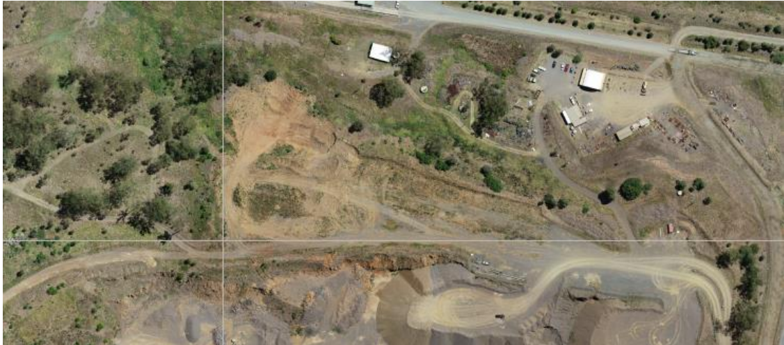
Plate 9: March 2023 Overburden area Aerial Image
