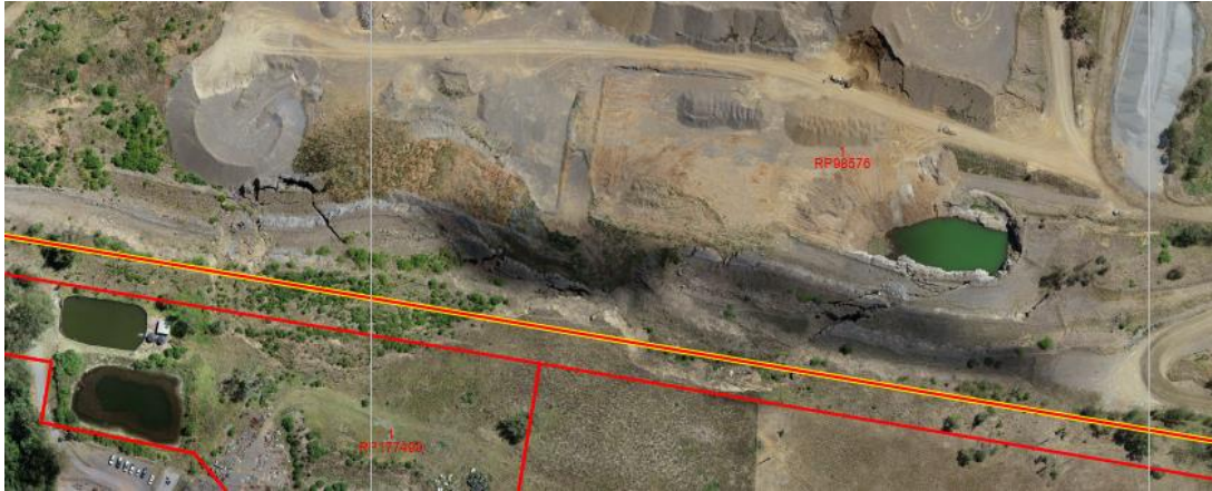
Plate 7: March 2023 Landslip Aerial Image
