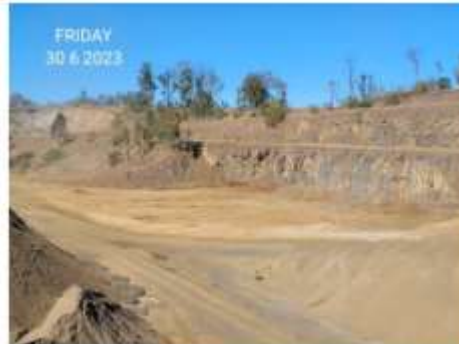
June 2023 – West Pit fill complete (looking east)
