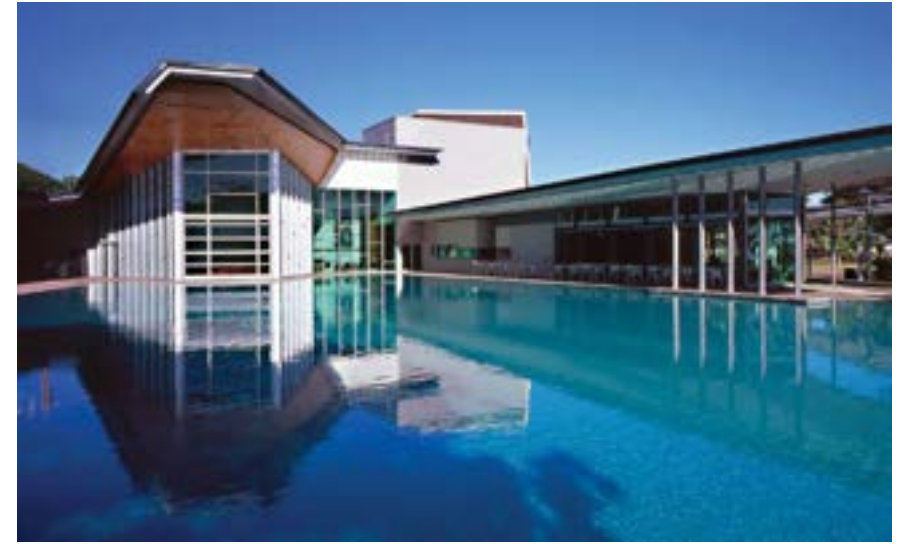
Riverway Cultural Centre & Lagoons - Townsville
