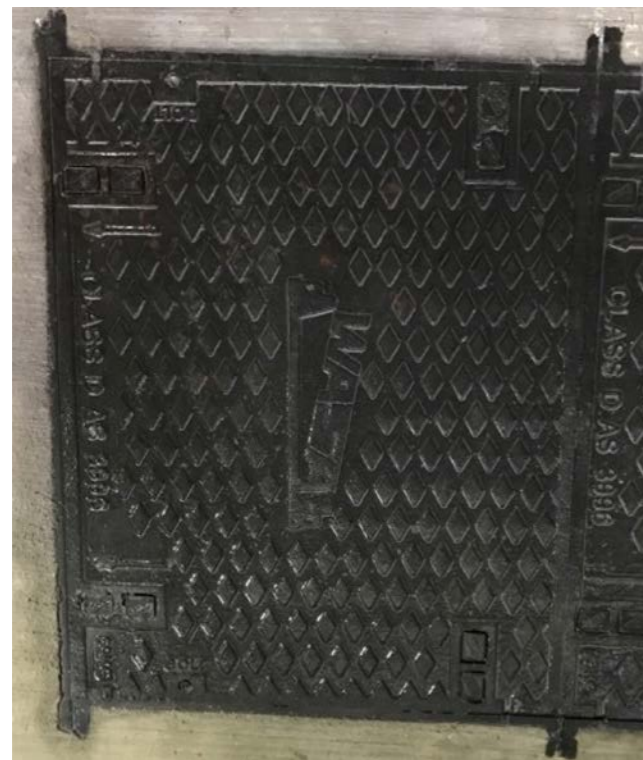
TYPICAL CAST IRON COVER
