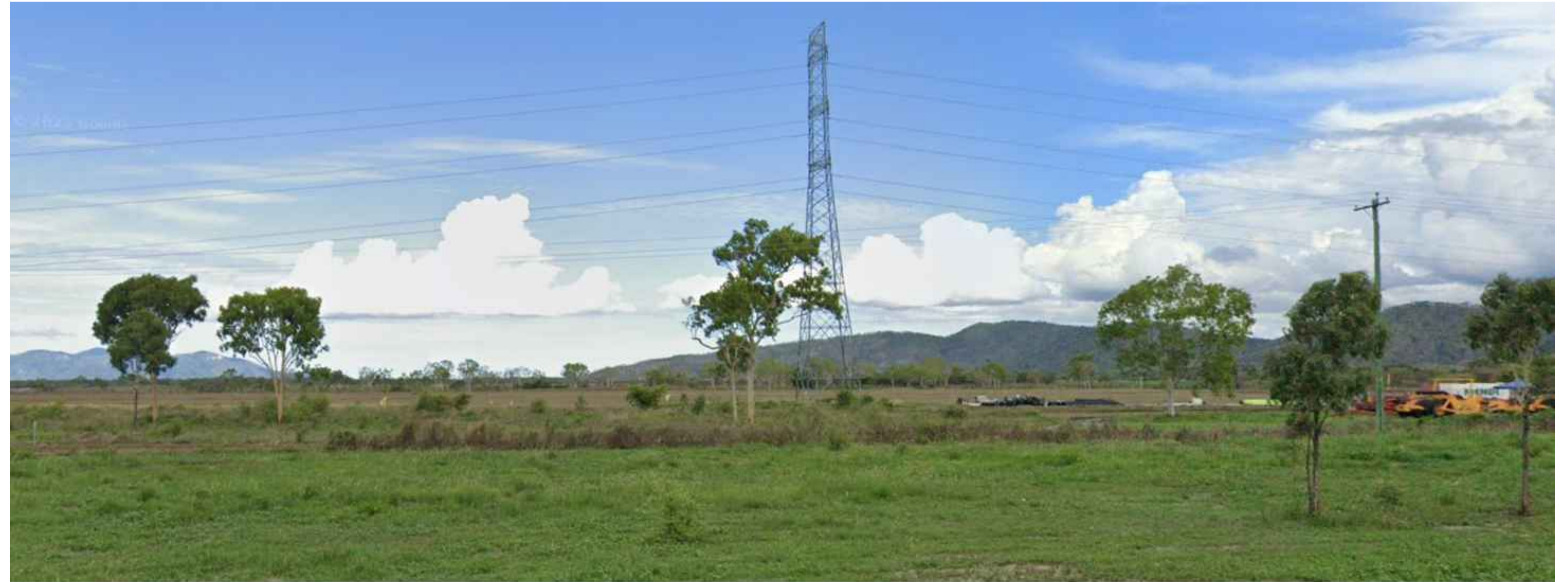
V1 - RON McCLEAN DRIVE LOOKING SOUTH-EAST (ACROSS HIGH VOLTAGE POWER LINE CORRIDOR)
