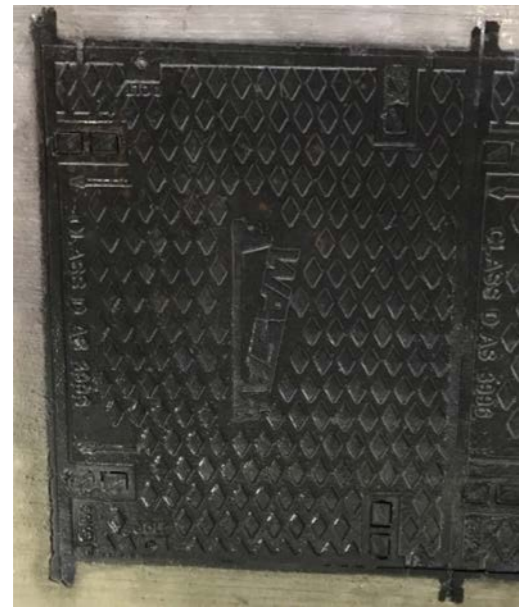
TYPICAL CAST IRON COVER
